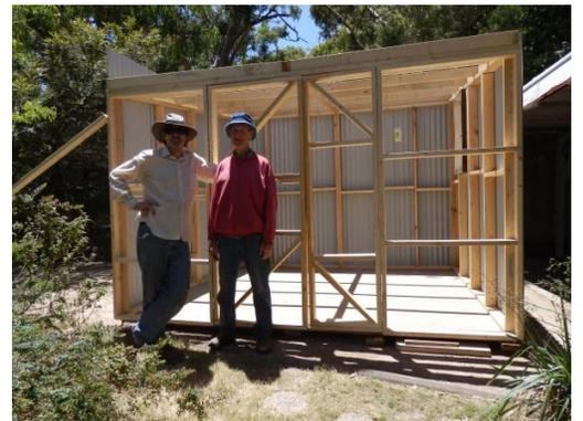
building was constructed in sections at a committee member's property over a period of weeks. The sections were then assembled to ensure that the building panels fitted together correctly. It was then disassembled and transported by ute and trailer to the carer's property. The sloping site was levelled and the flooring and wall and roof sections were then assembled on site by 3 volunteers in a day. Peter Cooper oversaw and
