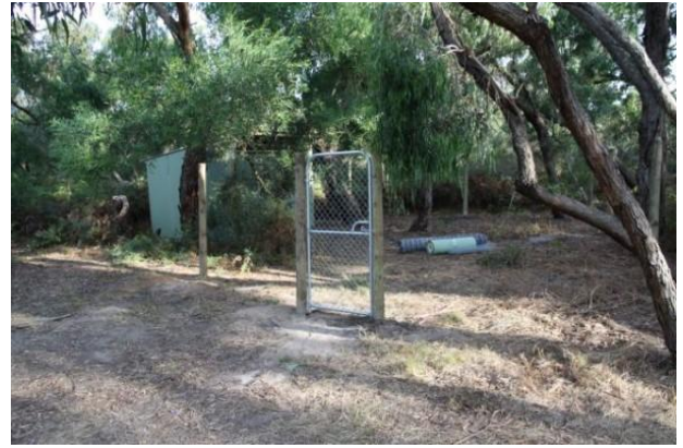
The roo compound under construction.
